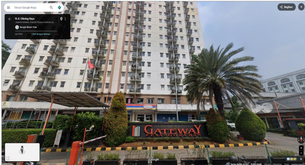
Figure 1. Location and Appearance of the Apartment Building
