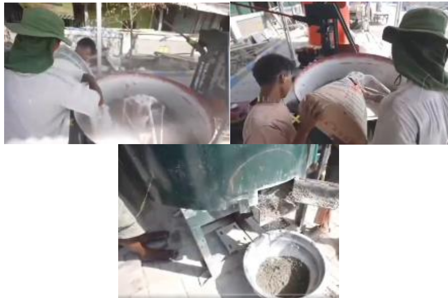
Figure 5. Concrete Mixing Process Source: Research Team Documentation, 2025
