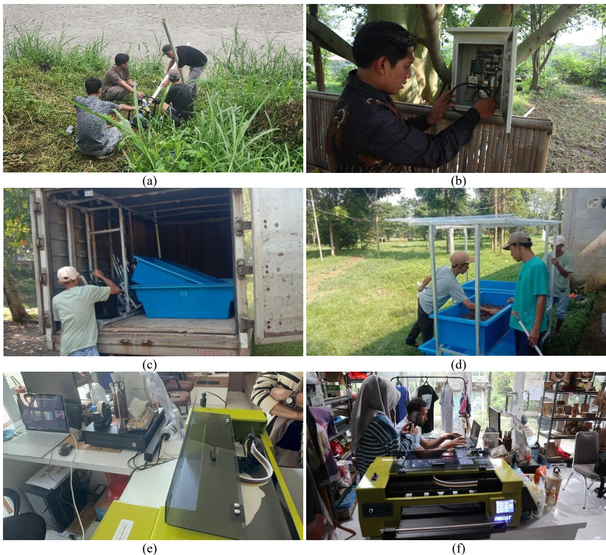
Figure 2. Technology Installation Stage, (a) Installation of pump to get the water from the river, (b) Installation of IoT, (c) The components of aquaponics, (d) Installation of Aquaponics, (e) Installation of DTF, (f) Setting of DTF
