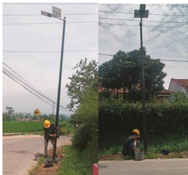
Figure 3. Installation of solar-powered public streetlight
